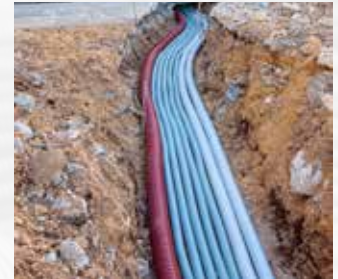
LFMC and LFNC protect wiring in Direct Burial
