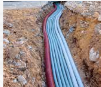
LFMC and LFNC protect wiring in Direct Burial
